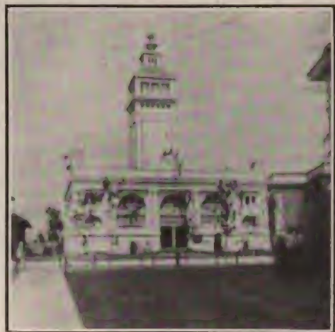
THE SAN FRANCISCO BUILDING
